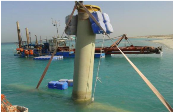
Intake Pipes Installation
